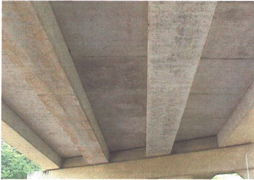
BOTTOM OF DECK
