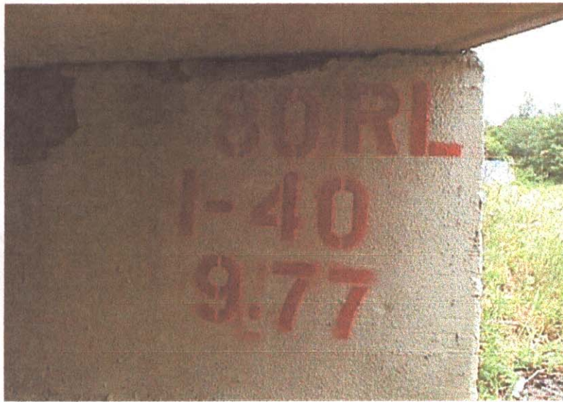
BRIDGE NO. AT ABUTMENT # 1
