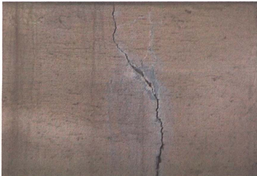
ABUTMENT #2 CRACK
