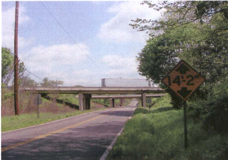
RIGHT SIDE VIEW W/CLEARANCE SIGN 14' 2"
