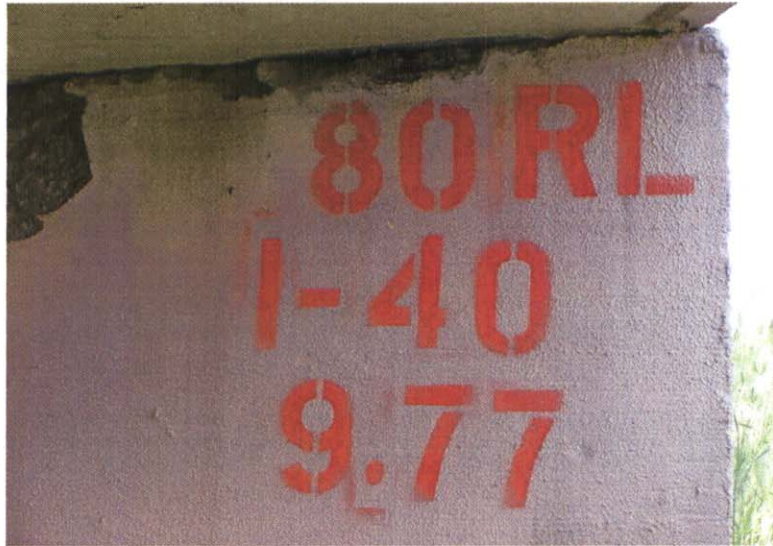
BRIDGE NO. AT ABUTMENT # 1
